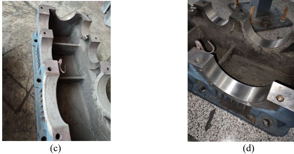
Fig.3 (Cont.). Metal spray welding process: a) Undercutting, b) Metal spraying, c) Welded area, d) Final area (after final machining)
